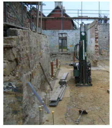
We operate variety of modular drilling equipment to enable ground investigation in restricted access environments, where conventional equipment cannot be mobilised and it would otherwise be difficult to obtain samples or carry out testing. This includes existing basements, lightwells, buildings, low headroom areas, close-up against walls, in rear gardens and on steep slopes. The equipment will generally pass through a standard domestic doorway.
