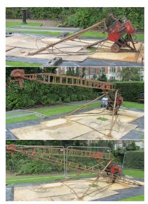
Often site investigation work requires sampling and testing to be conducted in restricted and/or confined access environments with limited headroom. This is particularly problematic for deeper boreholes as the equipment traditionally used tends to be rather
