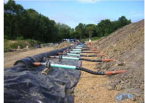
Figure 9 - Reactive Barrier Wall Installation
