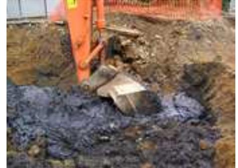
Figure 4 – Stabilisation to aid Excavation
