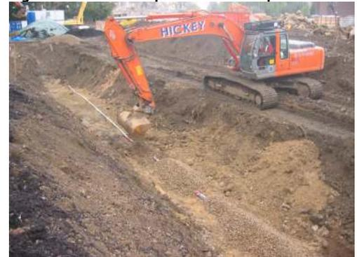
Figure 9 – Below ground (In-situ) Biopile
