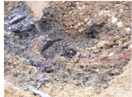
Figure 3 - Zonal Excavation and Remediation
