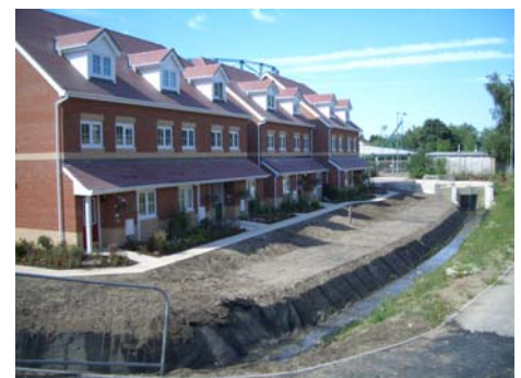
Figure 8 – Phase 2a Complete. Barrier wall beneath footpath and new stream channel
