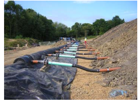
Figure 7 – Reactive Barrier Wall Installation
