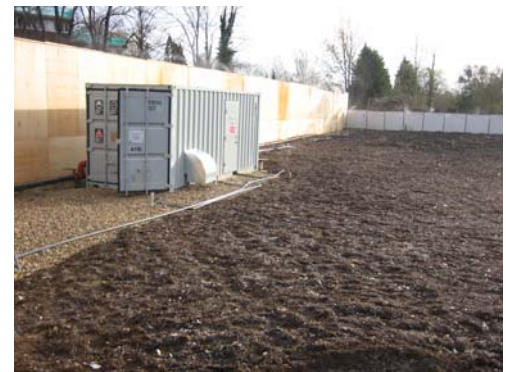
Figure 10 – Insitu Treatment Gasholders
