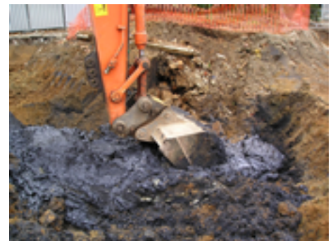
Figure 3 – Excavation of Tar Tank Structure
