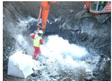
Figure 4 – Stabilisation to aid Excavation
